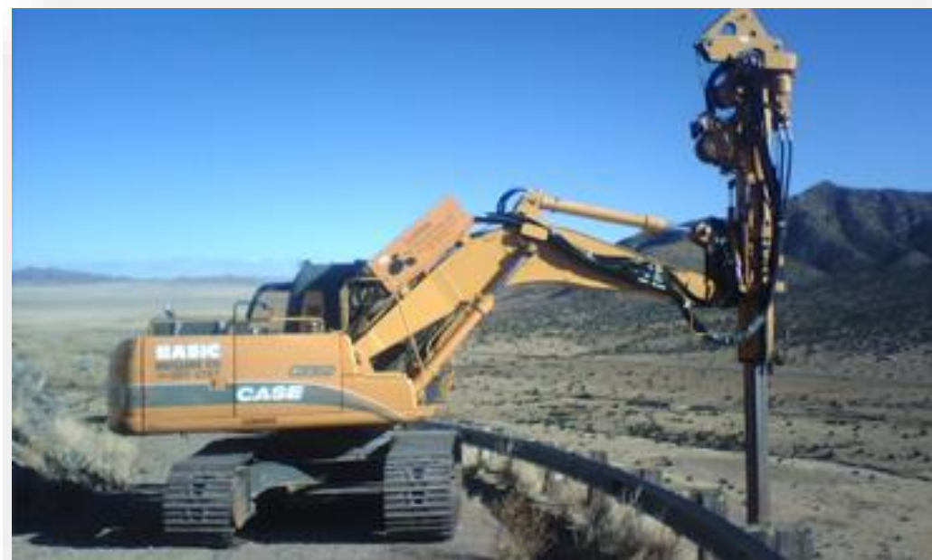
Foundation Drilling
