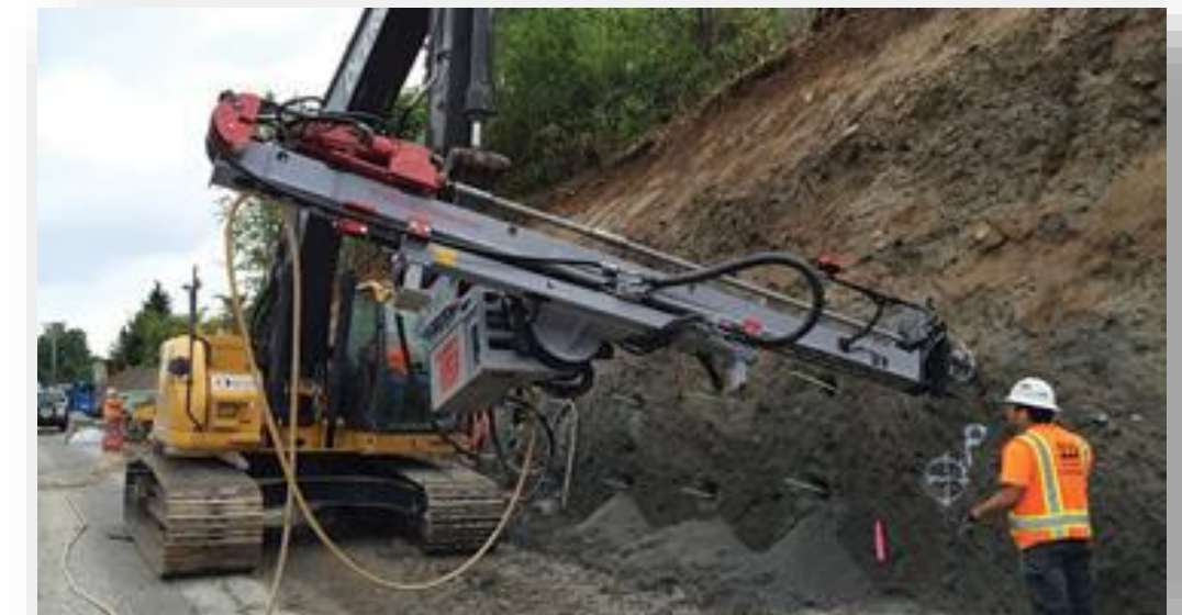
Geotechnical Drilling
