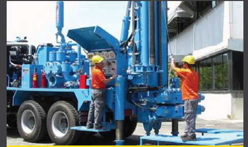
Water Well Drilling
