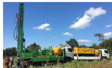
Water well drilling
